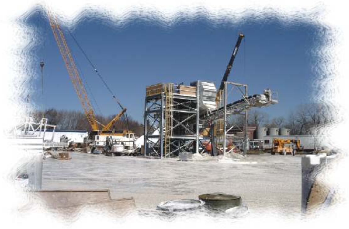
Northwest Side Relief Sewer at County Grounds
