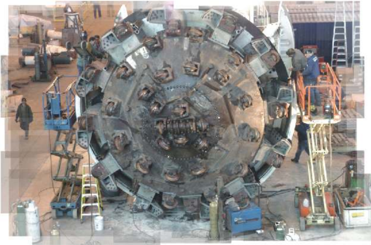
Tunnel Boring Machine - Northwest Side Relief Sewer
